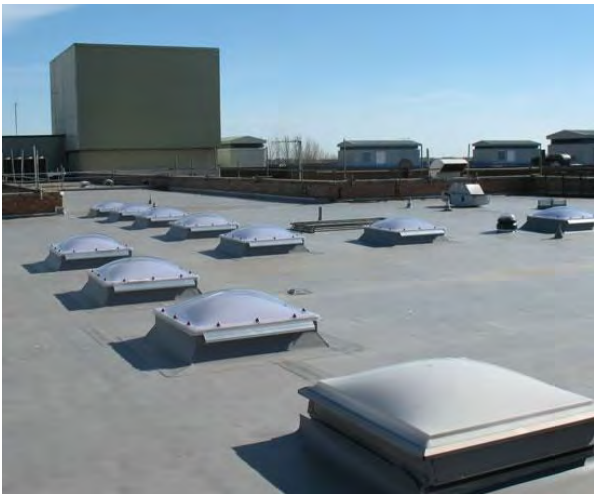
Single ply membrane roof and roof lights
