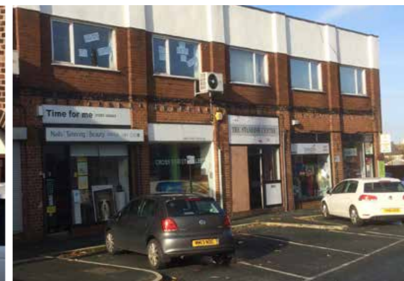
POOR QUALITY FRONTAGES AT THE STANDISH CENTRE
