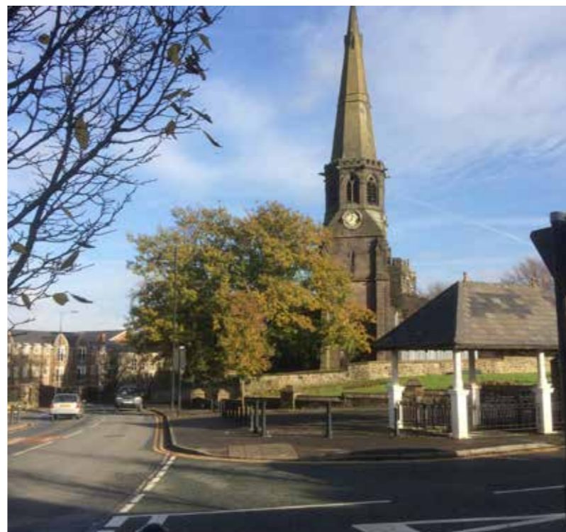
EXISTING TARMAC SURFACING FRONTING THE HISTORIC SQUARE
